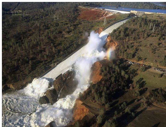
Flooding events threaten lives, property and infrastructure. The Oroville Dam where the main spillway eroded after the reservoir rose 50 feet in a few days, is an example of the effects.
