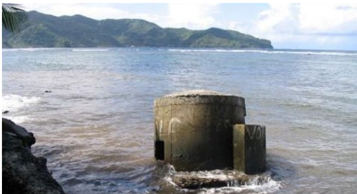
Figure S.MH.14.5. WWII pillbox defensive structures are located along the shorelines of Tutuila, slowly being impacted by coastal erosion. (Photo Hans van Tilburg/NOAA)
