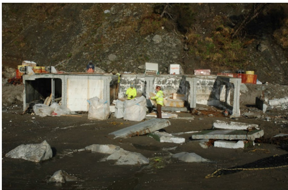
Figure R.4 Salvage status of dock from the Japanese tsunami on March 21, 2013: 87% foam, and 25% concrete removed by helicopter. Photo: OCNMS.
