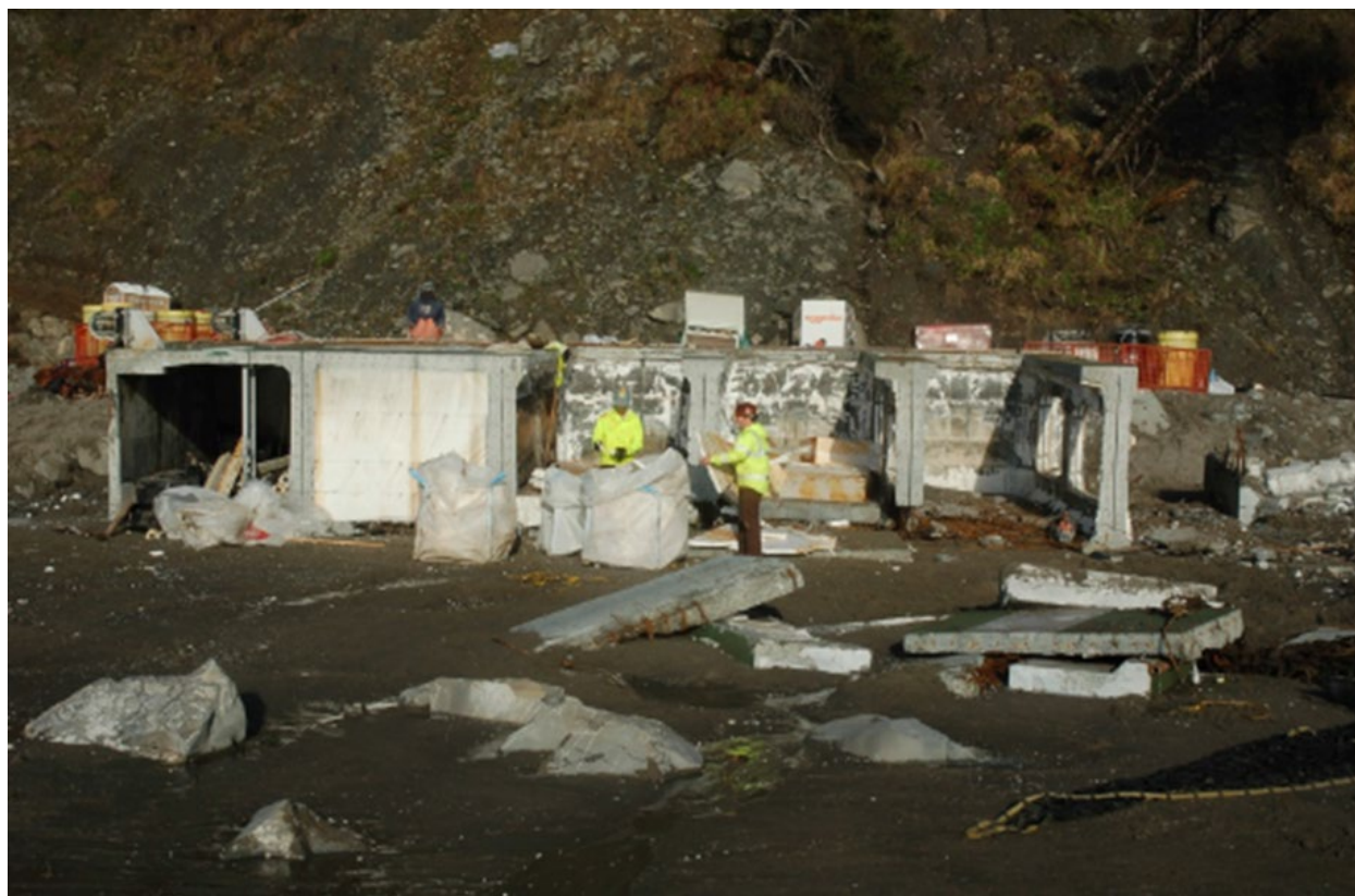
Figure R.4 Salvage status of dock from the Japanese tsunami on March 21, 2013: 87% foam, and 25% concrete removed by helicopter. Photo: OCNMS.
