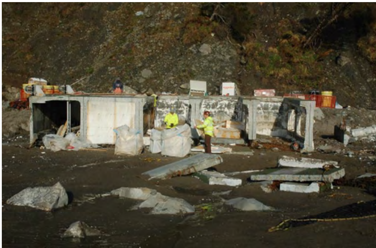
Figure R.4. A dock dislodged during the Japan tsunami, washed ashore in Washington. As of the date of the photo (March 21, 2013), 87% of foam and 25% of concrete had been removed by helicopter. Photo: NOAA
